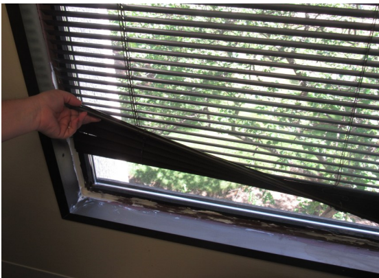
Caulk repairs for leaking windows
