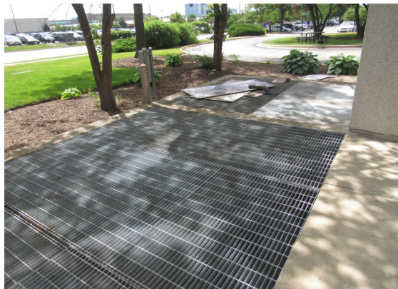
Exterior access to generator/tunnel
